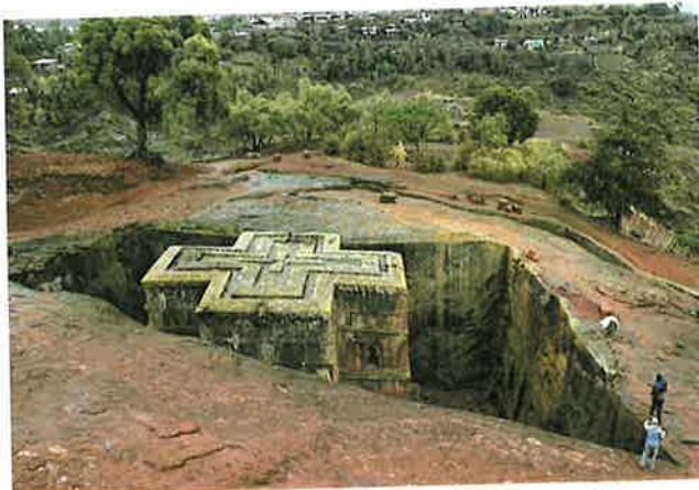
2.14 St George's church in Lalibela, Ethiopia, is a rock-hewn building, created by excavation from the surrounding stone.
